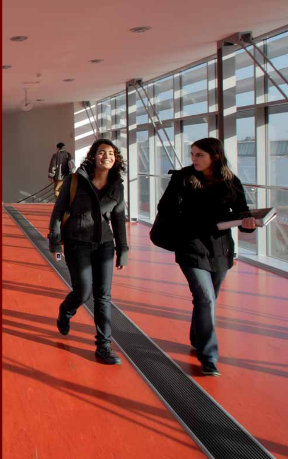
Leading lines in hallways are designed to help students with impaired vision
